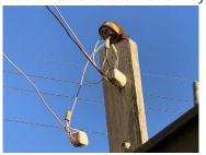
19. Service: Copper - Service wires spliced in panel box. Should be continuous from the service drop to the panel. Recommend further review by Electrician and repairs as needed.
