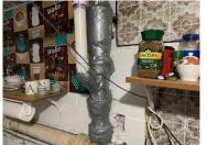
30. Faucets/Traps: Marginal - Kitchen sink faucet hot/cold reversed. Kitchen sink drain should be "P" trap. Previous repairs to kitchen sink drain. Tub spigot loose and not flush with the wall in front bath. Tub drains slow in front bath. Have checked.
