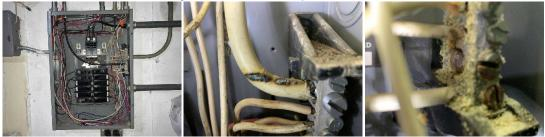
23. Basement Electric Panel Breakers: Marginal - Multiple double tap breakers in panel. No open positions. Recommend further review by Electrician and repairs as needed.
