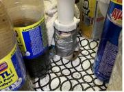
31. Sump Pump: Submerged - Recommend battery back up for sump. Could not determine sump discharge location.
